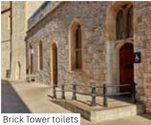
Brick Tower toilets
